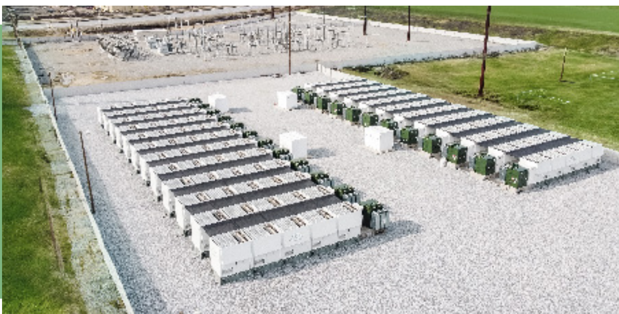
This 48 MW microgrid installation for the California Department of Water Resources features 120 natural gas generators that provide fast-response dispatchable capacity to the grid during peak load shortfall.
