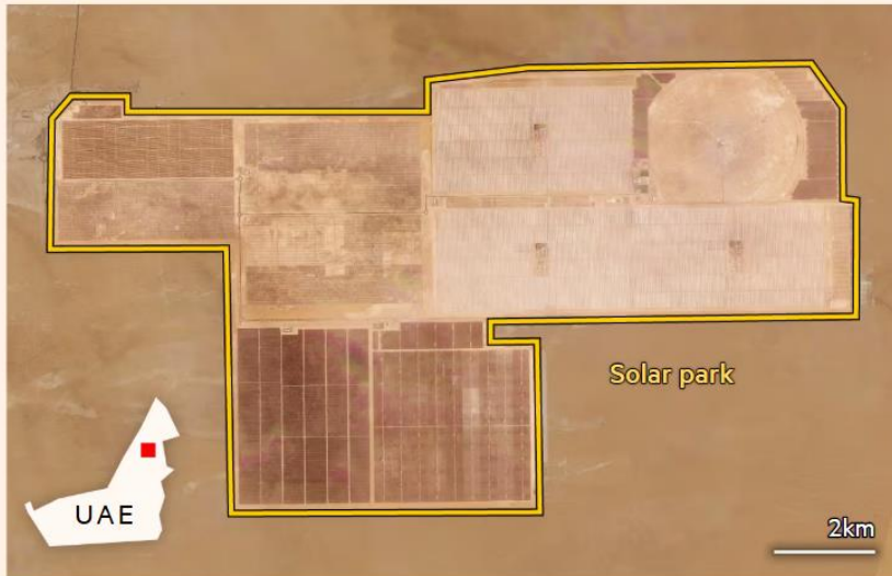
Chinese companies are playing a growing role in clean energy developments in the Gulf region, including at the Mohammed Bin Rashid Al Maktoum solar park in Dubai. The megaproject is one of the largest solar farms in the world, with a planned capacity of 7.2GW by 2030.
